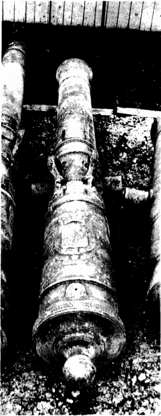
Figure 14. Brass 6-pounder, cast by the Verbruggens in 1774, weight: 19 hundredweight 2 quarters 6 pounds, length: 8 feet. (The Royal Artillery Institution, Woolwich, U.K., The Rotunda, II/59.)
